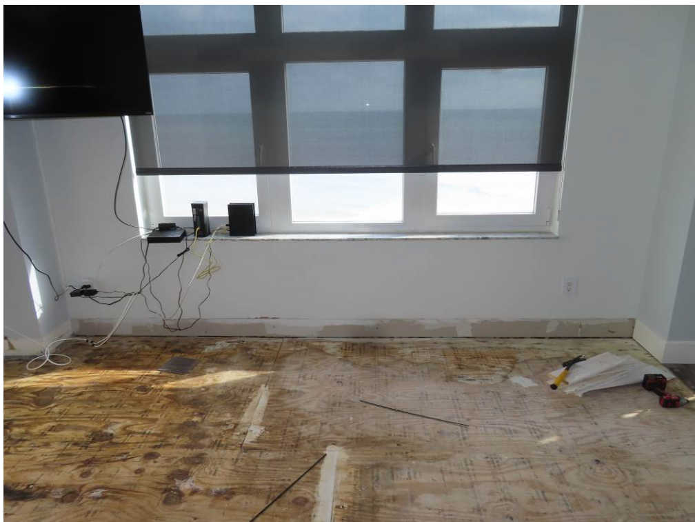
Photograph 2 Unit 406 Flooring Removed and Subfloor Staining under Windows
