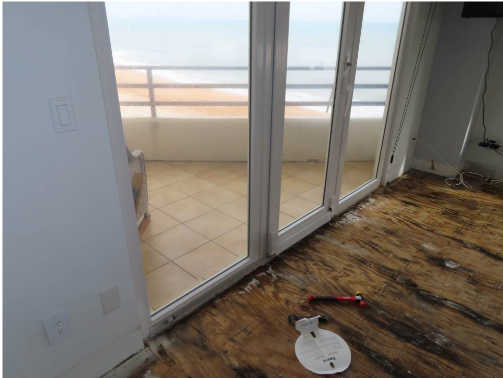
Photograph 1 Unit 406 Flooring Removed and Subfloor Staining at Sliding Door
