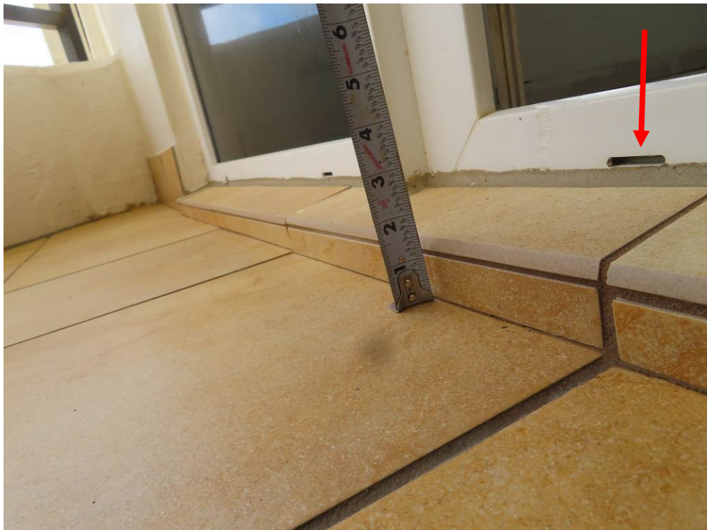
Photograph 6 Unit 406 Exterior Door Curb and Sealants, Door Weeps Remain Open
