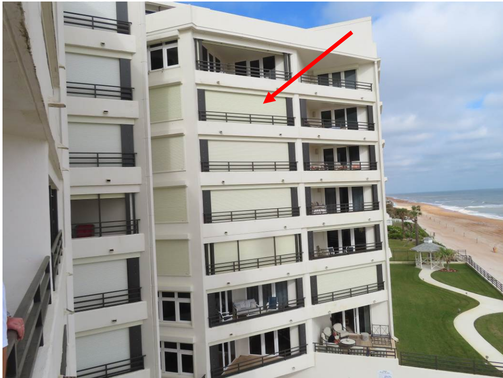
Photograph 7 Hurricane Shutters Installed on Multiple Units
