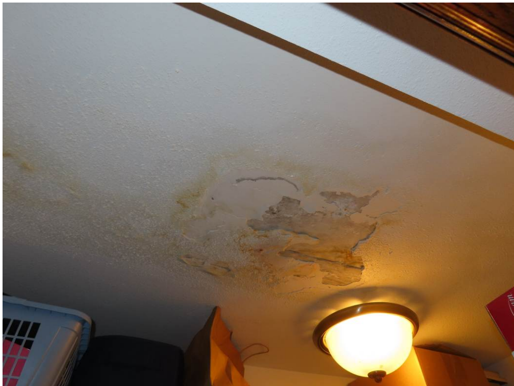
Photograph 8 Unit 706 First Unit Level Closet Ceiling Damage
