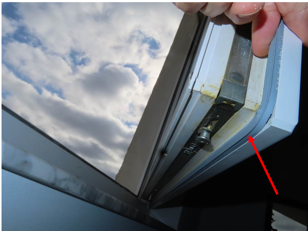
Photograph 4 406 Casement Window Inner Weather Stripping
