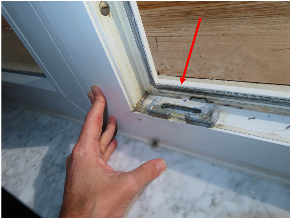
Photograph 3 406 Casement Window Outer Weather Stripping
