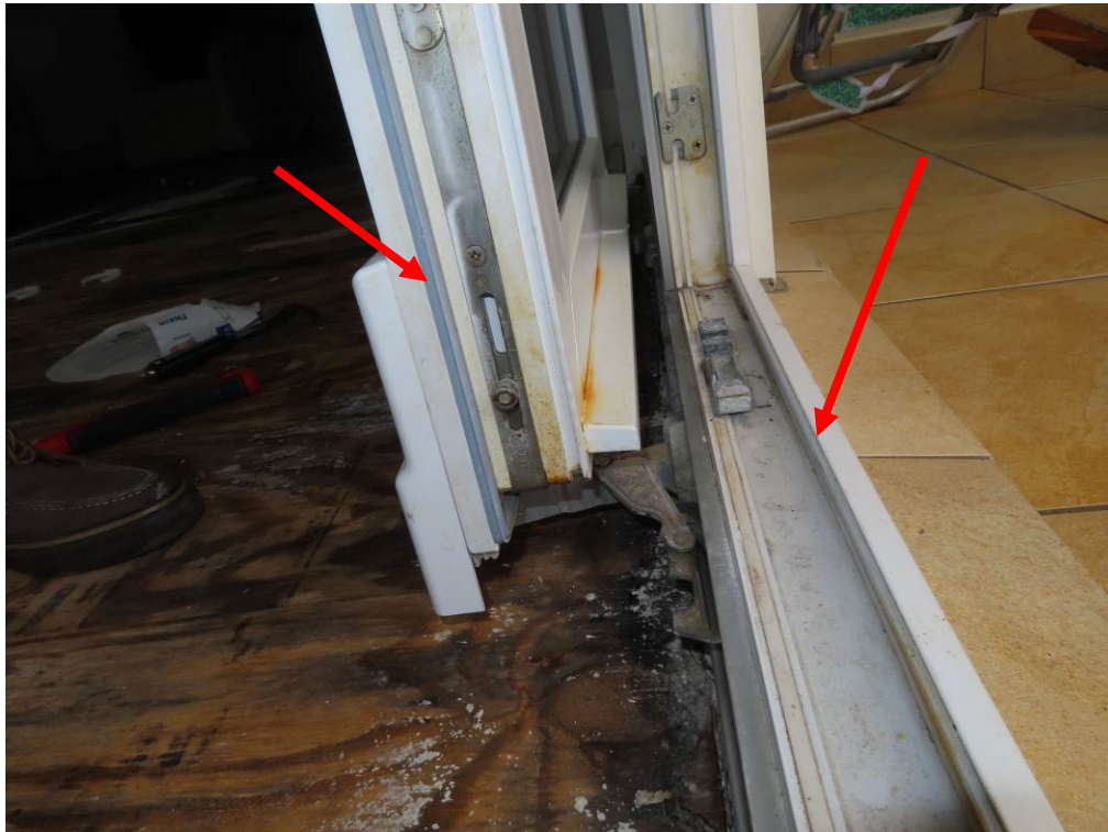
Photograph 5 Unit 406 Inner and Outer Weather Stripping Indicated
